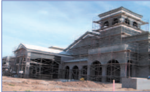
The $10 million Gilbert Emergency Hospital under construction
